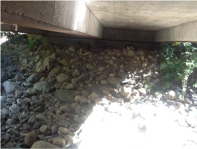
Right Bank Abutment when facing downstream
