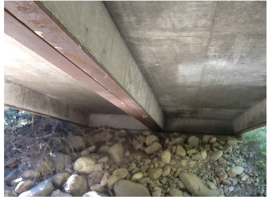
Underside of bridge
