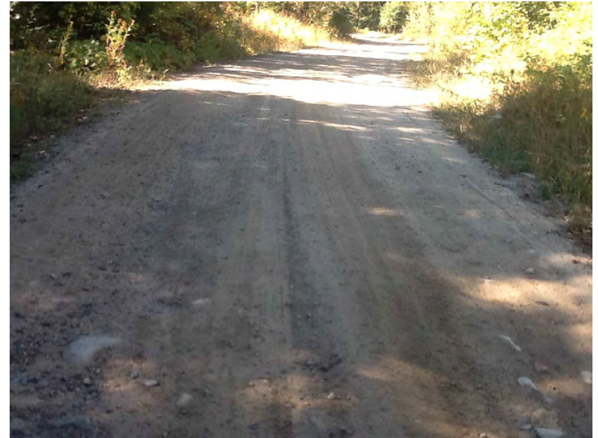
Left approach facing away from structure
