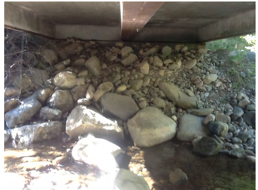
Left Bank Abutment when facing downstream
