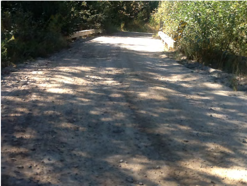
Right approach facing structure
